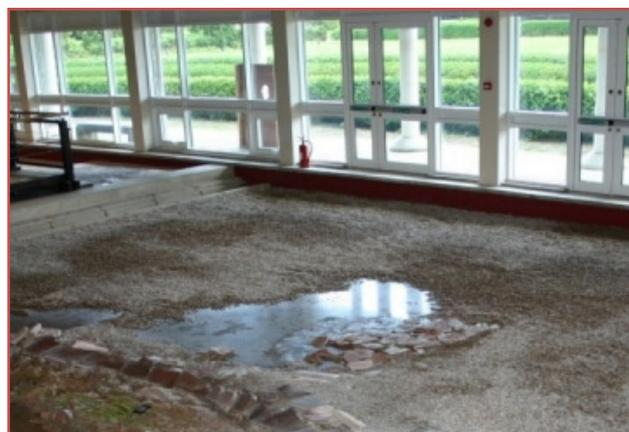
The mosaics in the North Wing of the Palace are under threat from flooding, temperature and humidity fluctuations, and algal growth. An 18 inch water main running just to the north has often caused flooding. It is now due to be moved or lined, which should remove the danger. The
