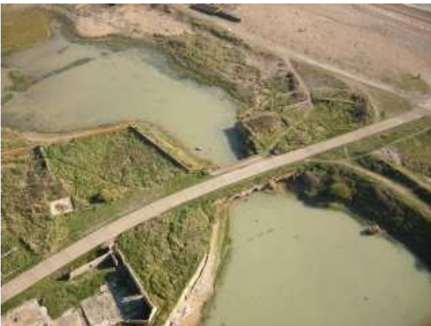
An aerial view of the site
