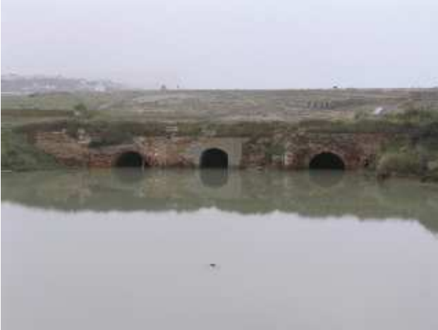
The tunnels under the bridge that fed the waterwheels
