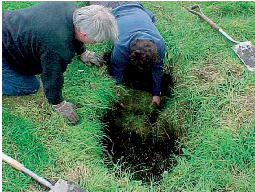
Removing the overhanging turf at the entrance to the subsided void
